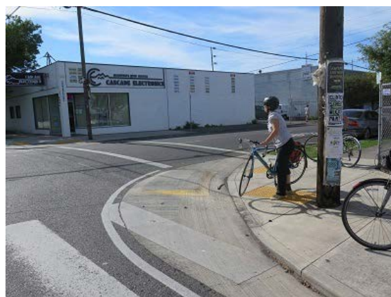
Figure 3-8: Truck Apron Helps Slow Turning Cars
