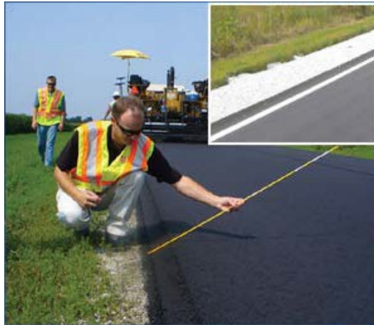
Figure 3-14: Photo Depicting "Safety Edge" Pavement Design
