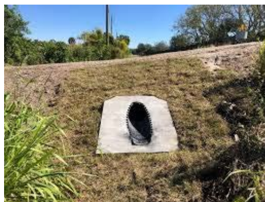
Figure 3-15: Mitered-End-Section Drain Pipe
