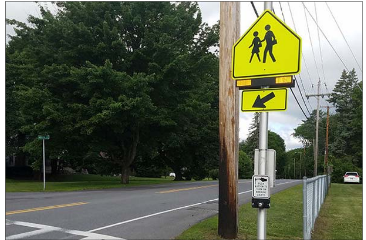
Figure 40. Rectangular Rapid Flashing Beacon (RRFB)
