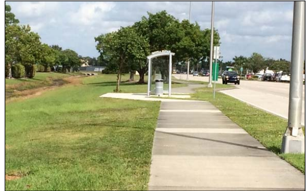
Figure 38. Sidepath on Airport Road
