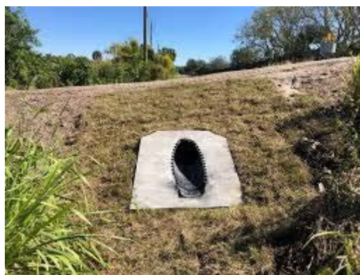
Figure 3-15: Mitered-End-Section Drain Pipe
