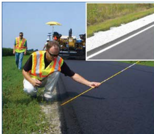
Figure 3-14: Photo Depicting "Safety Edge" Pavement Design
