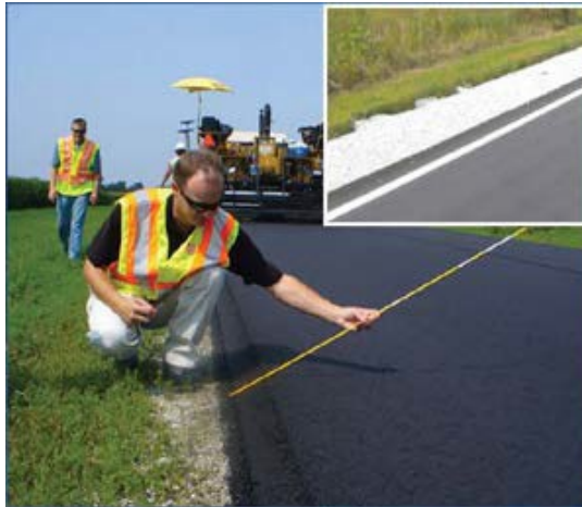
Figure 3-14: Photo Depicting "Safety Edge" Pavement Design
