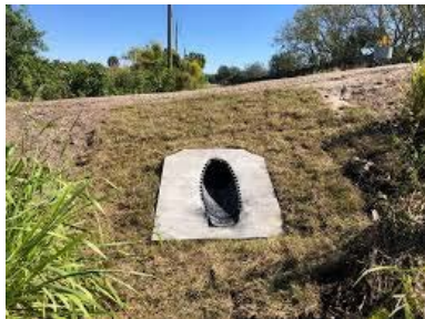
Figure 3-15: Mitered-End-Section Drain Pipe
