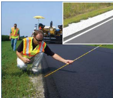
Figure 3-14: Photo Depicting "Safety Edge" Pavement Design
