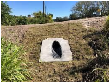
Figure 3-15: Mitered-End-Section Drain Pipe
