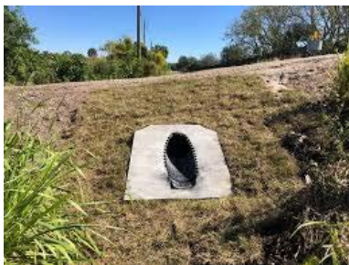
Figure 3-15: Mitered-End-Section Drain Pipe
