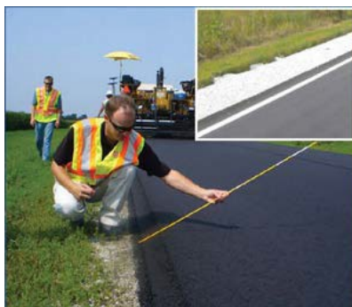
Figure 3-14: Photo Depicting "Safety Edge" Pavement Design
