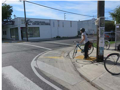
Figure 3-8: Truck Apron Helps Slow Turning Cars
