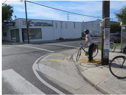
Figure 3-8: Truck Apron Helps Slow Turning Cars
