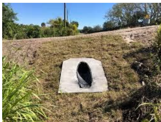
Figure 3-15: Mitered-End-Section Drain Pipe
