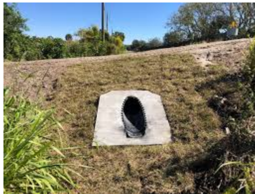
Figure 2-15: Mitered-End-Section Drain Pipe
