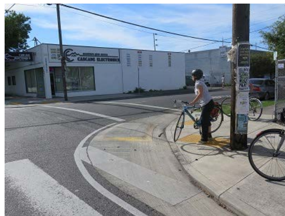
Figure 2-8: Truck Apron Helps Slow Turning Cars
