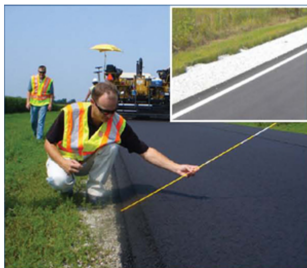
Figure 2-14: Photo Depicting "Safety Edge" Pavement Design
