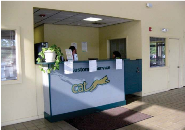
Incompliant desk height
