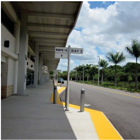
Looking North at the bus loading island
