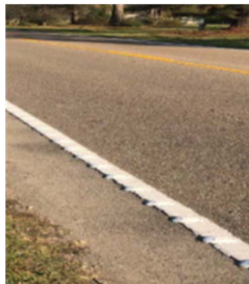
Figure 27. Audible Pavement Marking
