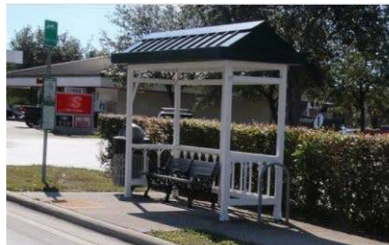
CAT shelter on Collier Boulevard
