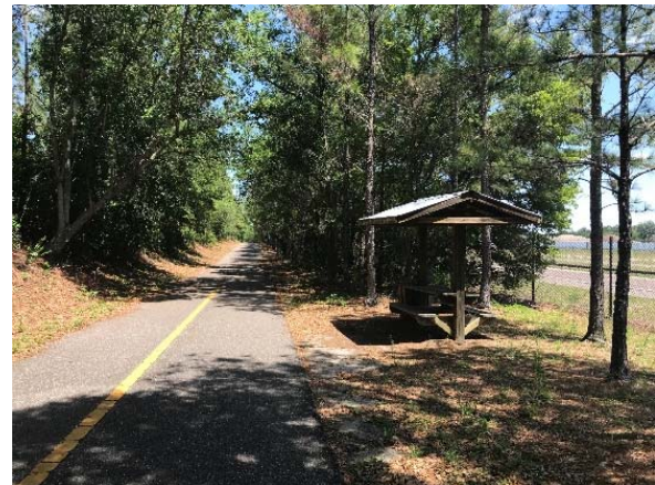
Figure 13: Shelter on Suncoast Trail
