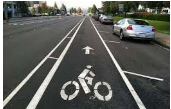
Figure 6: Buffered Bicycle Lane
