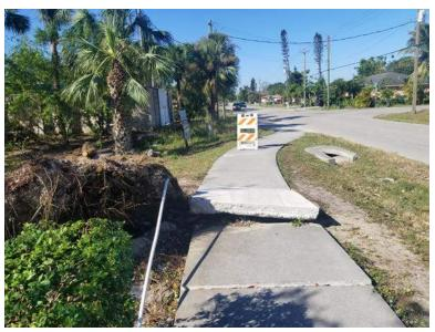
Figure 21. Sidewalks in Golden Gate City were impacted by Hurricane Irma in 2017.
