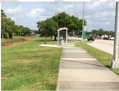
Sidepath on Airport Road adjacent to Naples Municipal Airport is a good example of a sidepath application that works due to the edge condition – the absence of multiple driveways and curb cuts. The Airport funded the bus. This short segment of Airport Rd is a good example of a Complete Street.
