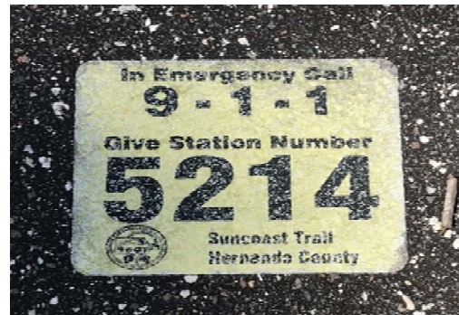
Figure 14: Embedded Pavement Decal
