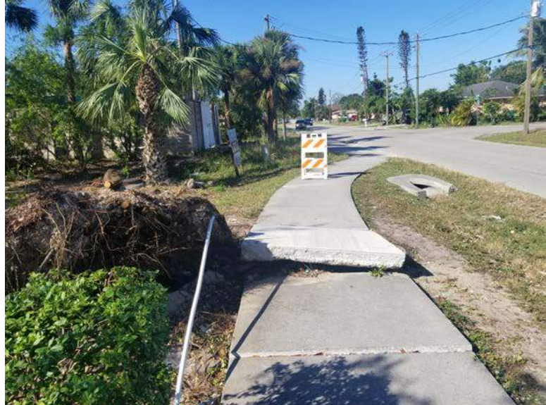
Figure 21. Sidewalks in Golden Gate City were impacted by Hurricane Irma in 2017.
